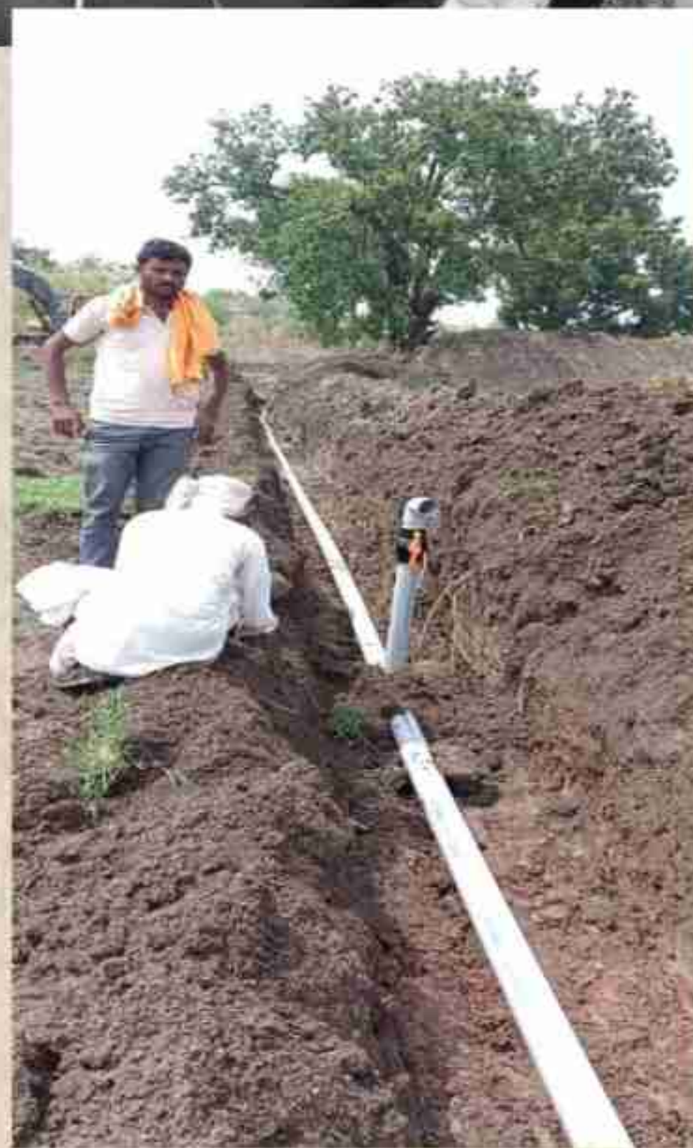
Constructed 2 Diversion-Based Irrigation (PHAD) Units Access for Farmers
